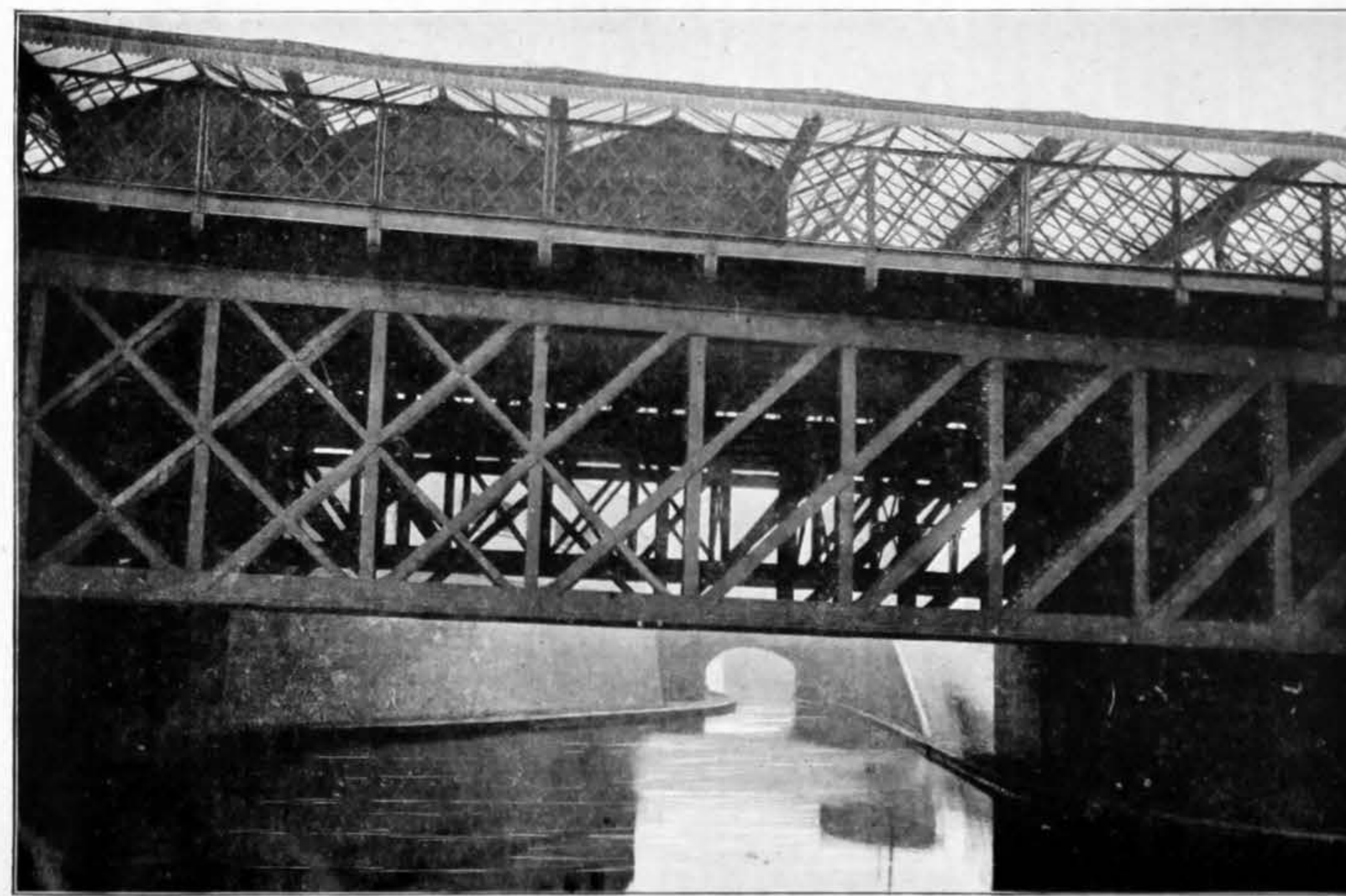
Fig. 3—PART OF GIRDER OVER CANAL BASIN
