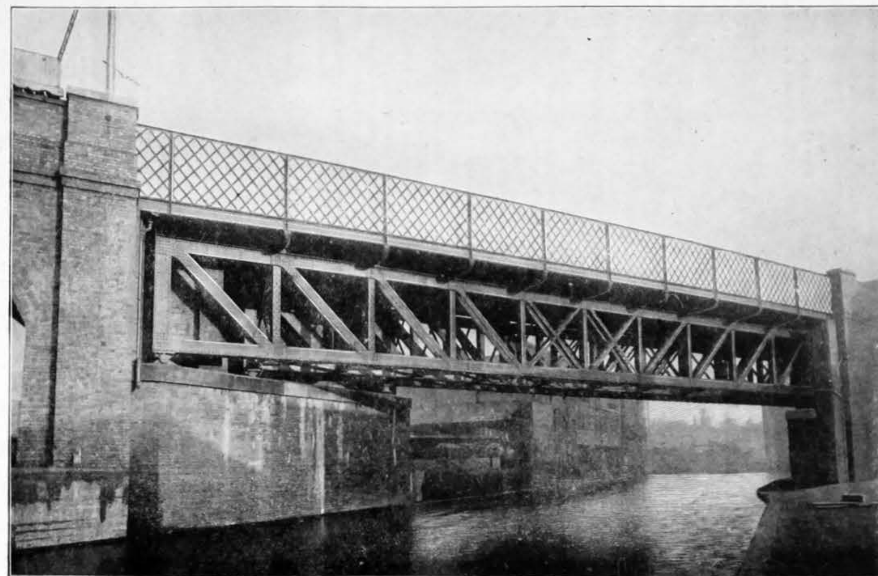
Fig. 4—BRIDGE OVER CANAL
