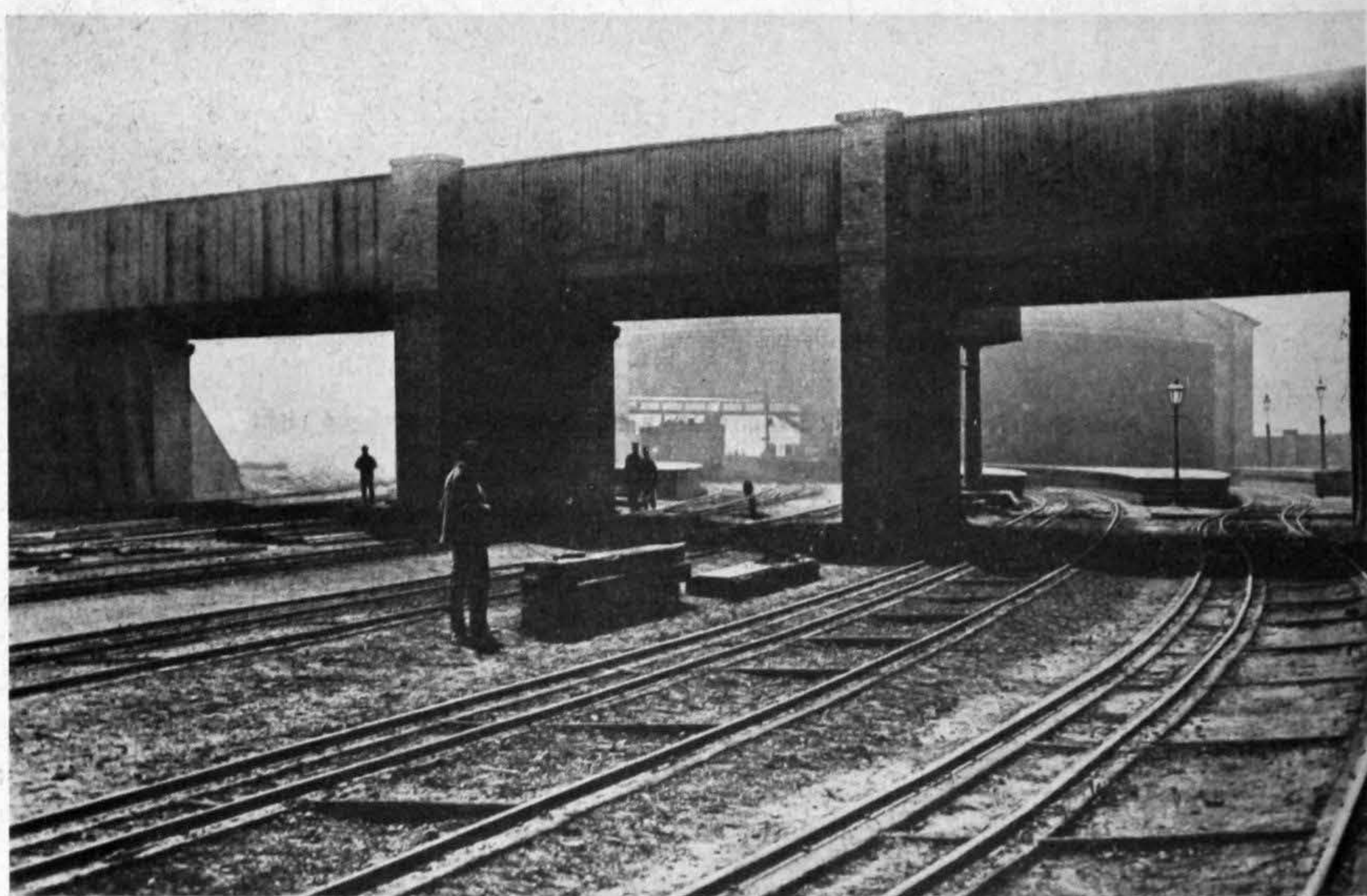
The north end of Wolverhampton low level station, G.W.R., in broad gauge days (about 1854), showing the third rail of the mixed gauge
