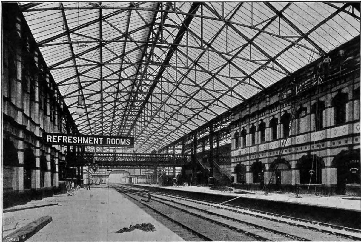
FIG. 55. VIEW OF INTERIOR OF STATION SHOWING MAIN SPAN.
